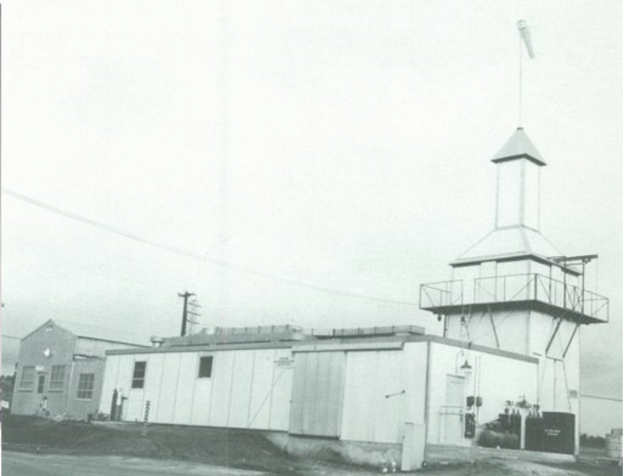
TINY TOWER—This 40-ft. instrumentation test tower, small in comparison to another AI tower of 102 feet, is used for sodium instrument tests. P. C. Borbon stands at the base.
