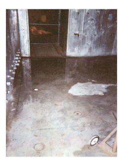
EPA needs to address the groundwater intrusion in Building 4024 (Left Photo). This is a reactor building with direct contact to the water table as groundwater finds a way into this vault area for decades now. This could be another source-point of Tritium in the groundwater aside from building 4010. If the Boeing Co. does not allow access into this structure for sampling of the groundwater, at depth sampling surrounding this former radiological facility should be considered.
