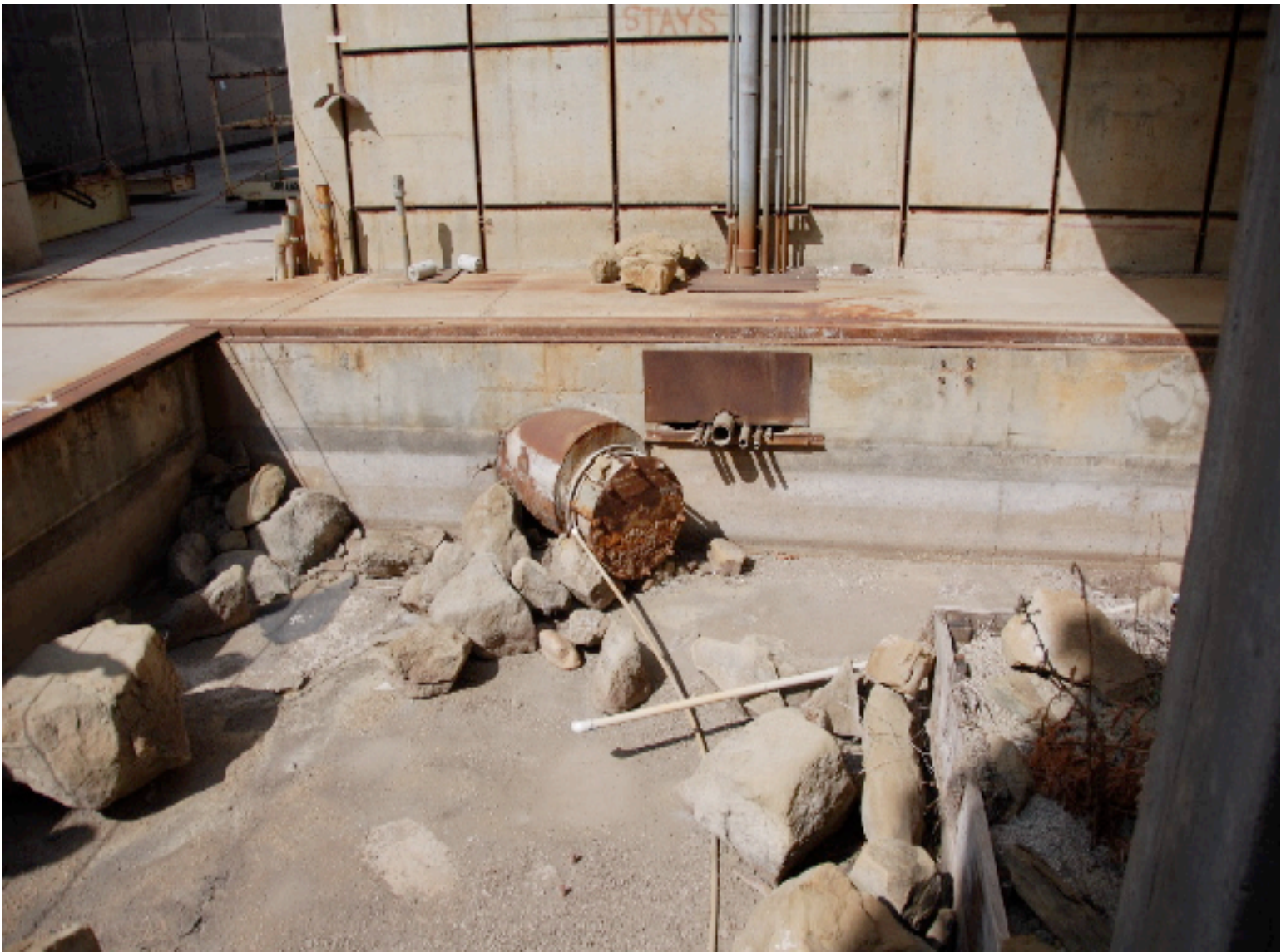
The above photos shows a test bay in the ELV/CTL II AREA that drains through the below pipe and into the burnoff pond seen in the middle and right photos.
