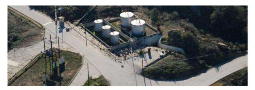
The photo above shows the ALFA/BRAVO Fuel Farm and as you can see the catch basin is designed to have runoff into the natural drainage that leads into the Storage Propellant Area (SPA) located in the NASA AREA II of the SSFL.
