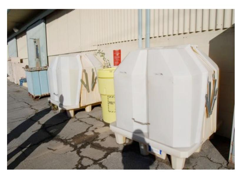
Areas around Building 204 in the NASA AREA II of the SSFL were used as staging and holding areas of solvents and other chemicals that impact the asphalt and then into the soil through cracks as seen in the photo above. This area sits high above other reporting areas and samples should be taken in logical step-out points from here on out.
