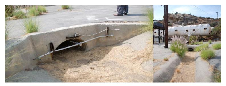
A spray system from the BRAVO LOX Tanks near WS-9 drain into a swale that leads into the drainage channel we saw above. These pipes are labeled Reclaimed Water and this area has historic documented contamination and should be looked into more thoroughly.
