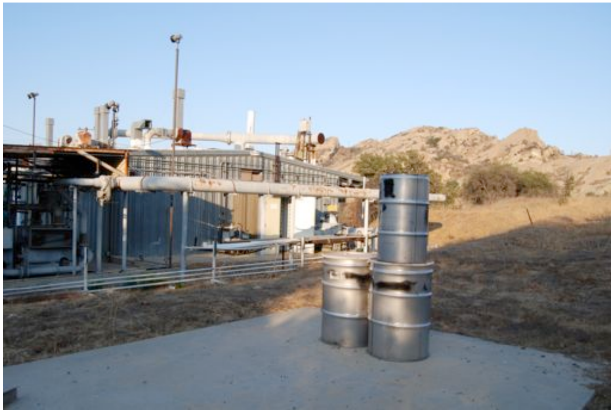
The above photo (Building 258 in AREA III) another example of the Concrete Pads in use.
