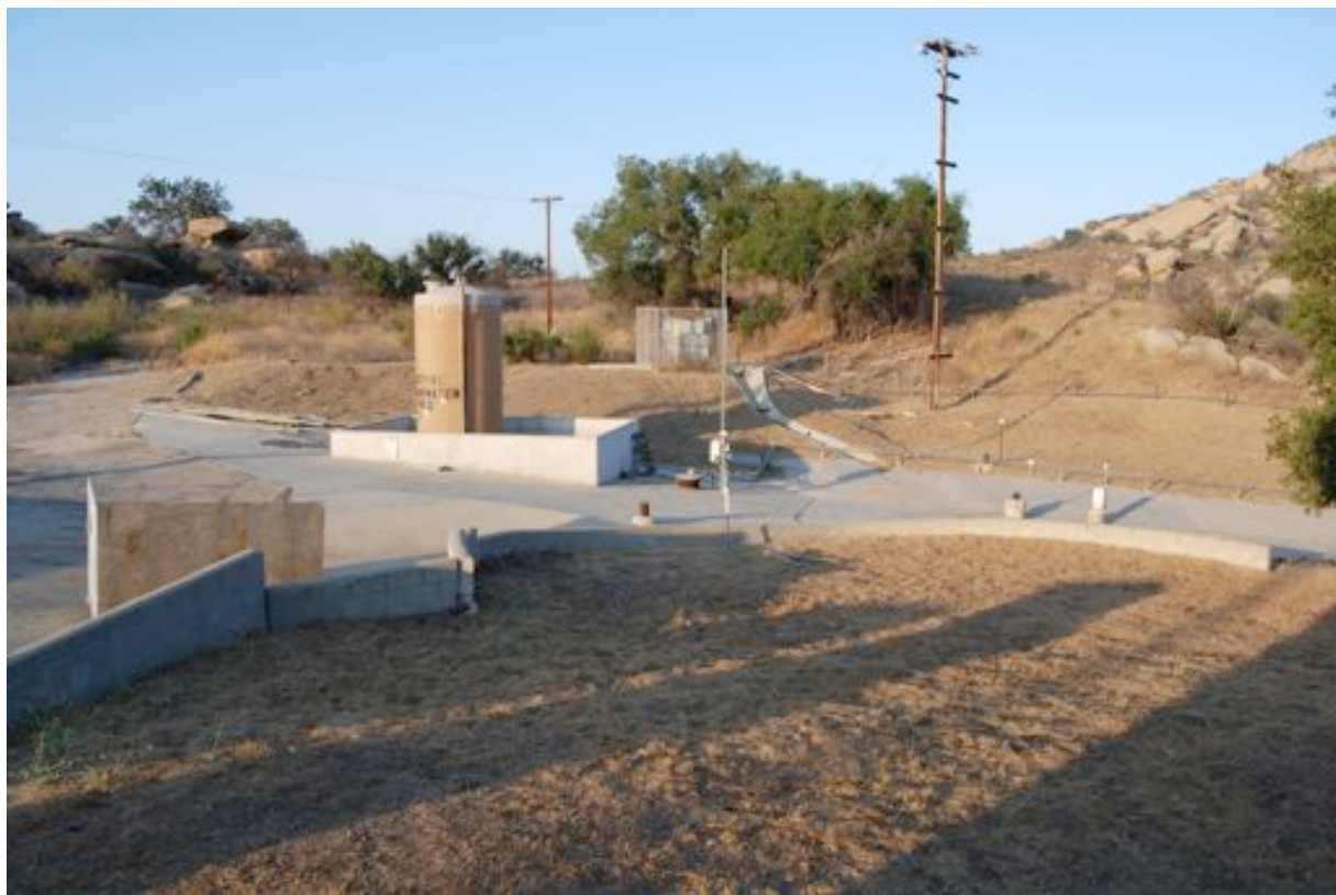
A portion of the Building 258 storm water runoff drains into the Silvernale Pond which overflows into the R-2 Pond and releases into the Los Angeles River via Bell Creek.
