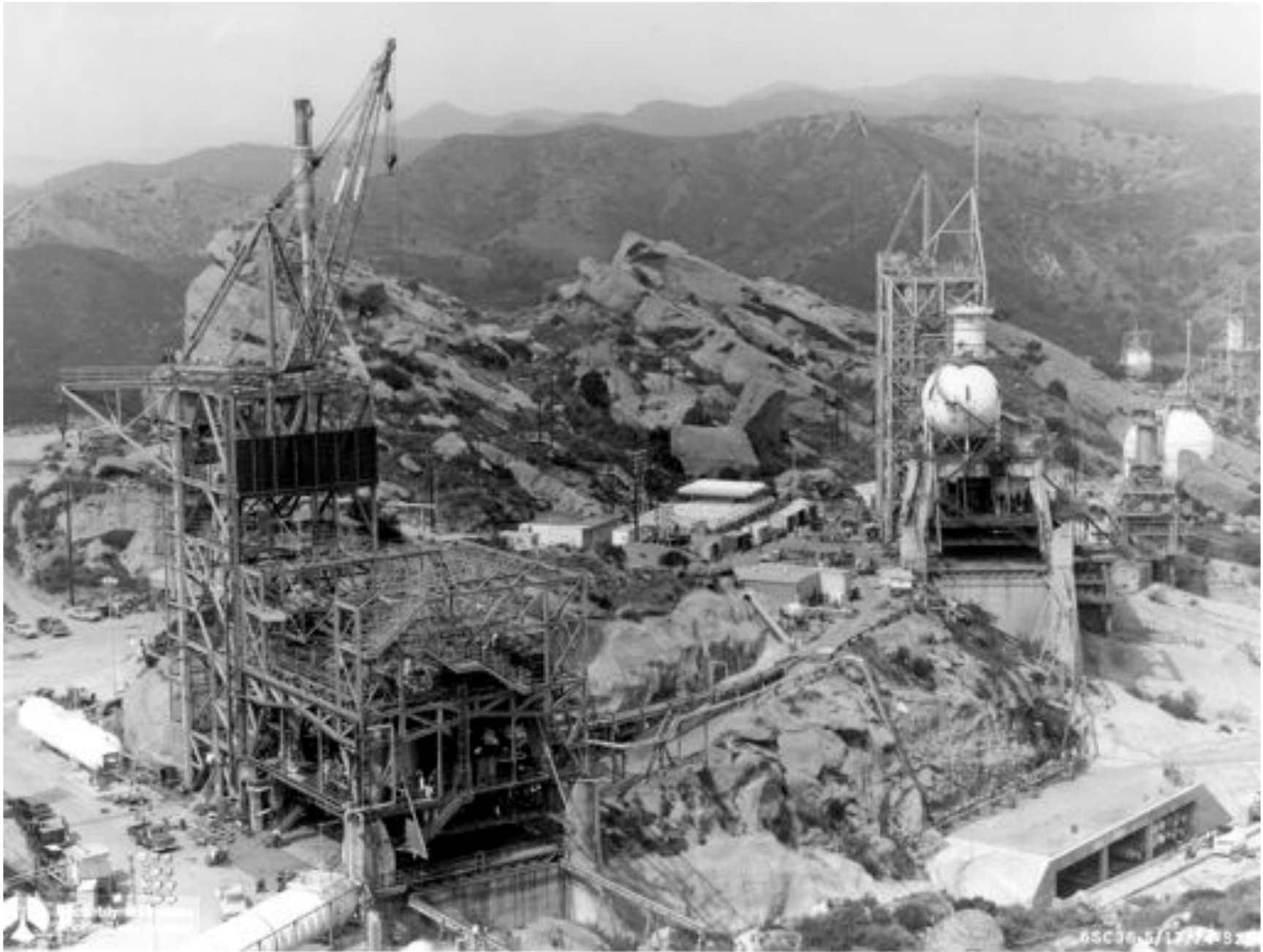
Coca Test Area Construction for SSME - 1974
