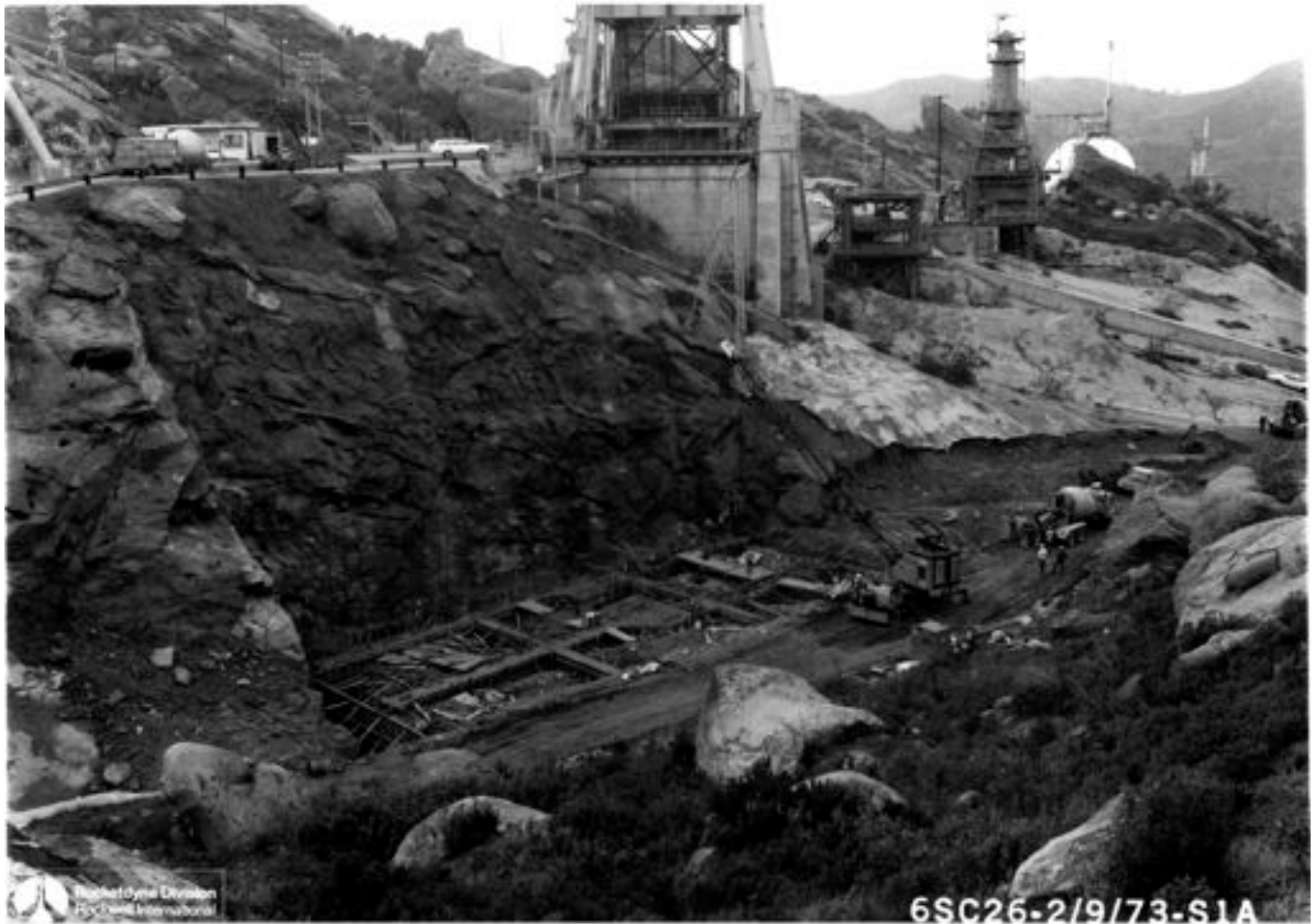
Coca Foundation Construction for "Vault" - 1973
