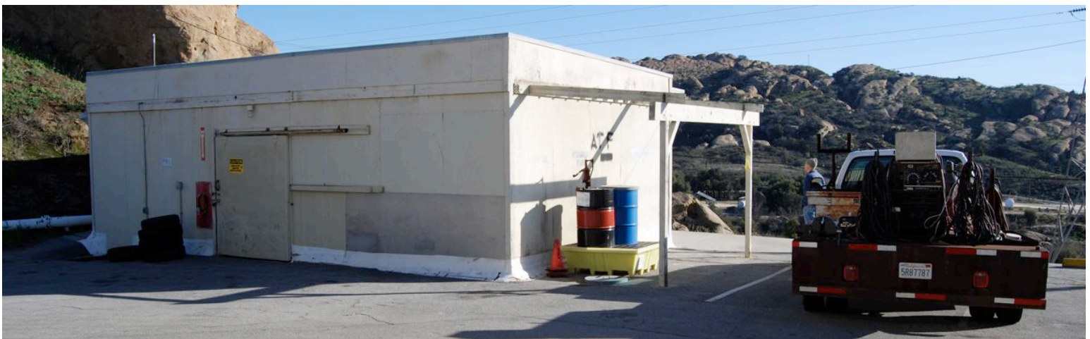
Building 2760 Prior to USEPA involvement
