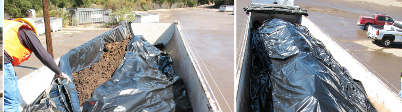
Soil is wrapped in plastic - "burrito wrapped" - and the bed of each truck is securely tarped.
