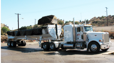
Soil removal from Outfall 8 is loaded into a lined transportation truck.
