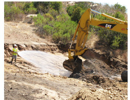
Soil removal at Outfall 8. Water is used as a dust control measure when soil is removed from the outfall and loaded into transportation trucks.
