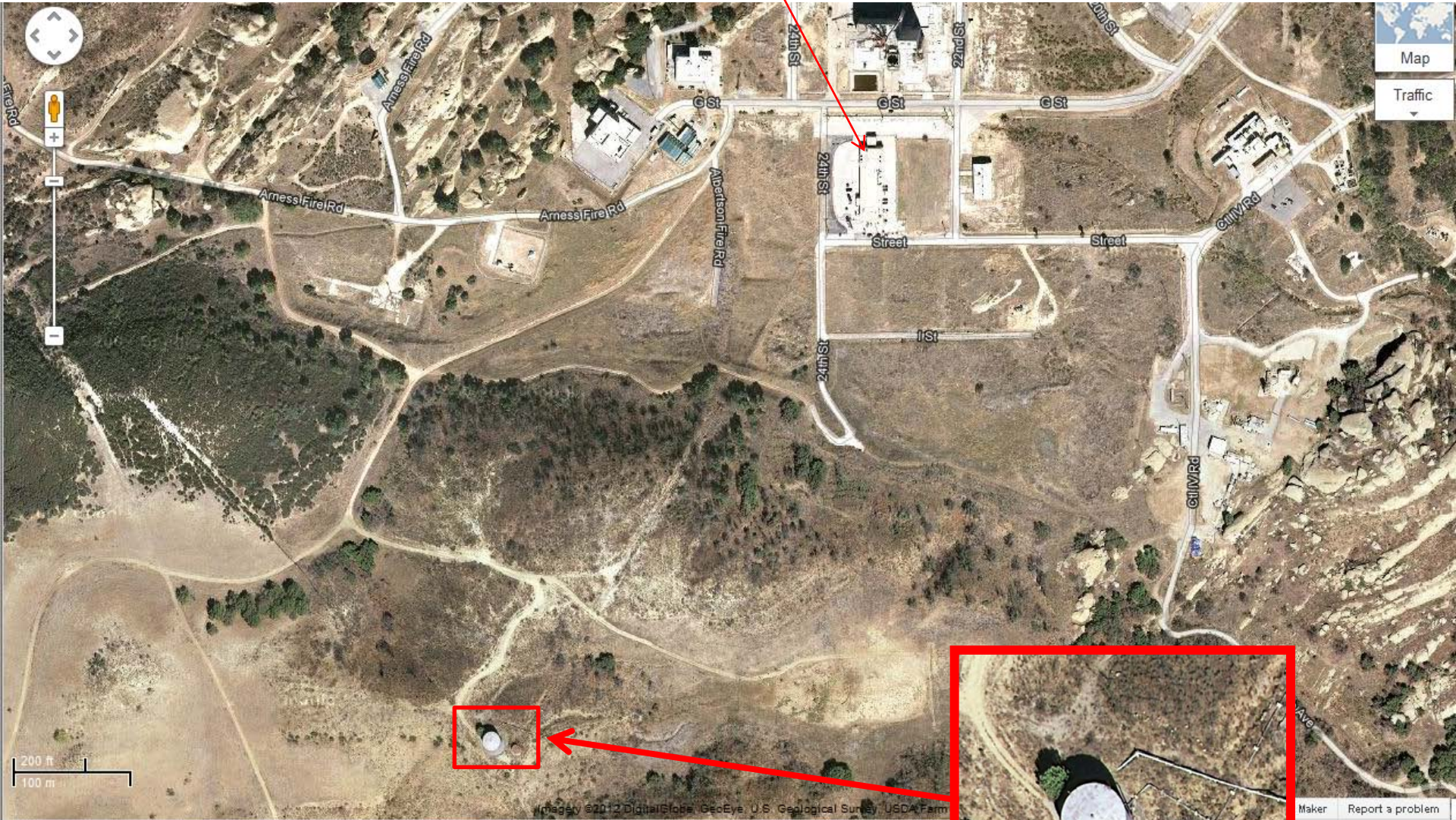
Area 4 Water tanks
