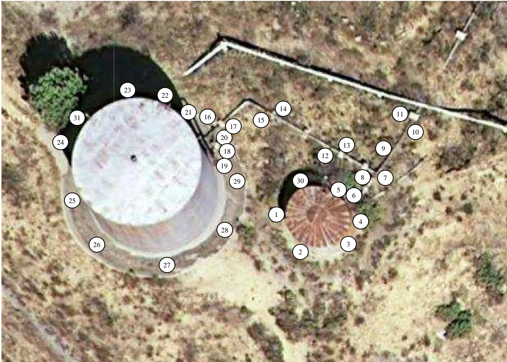
Area IV Site Water Tanks - Exterior Pre-Demolition Survey page 5 of 7
