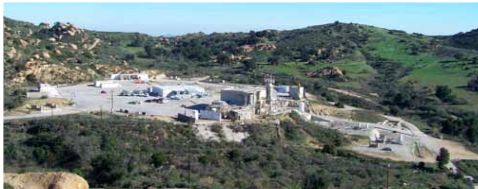
Before. Components Test Lab III before demolition.
