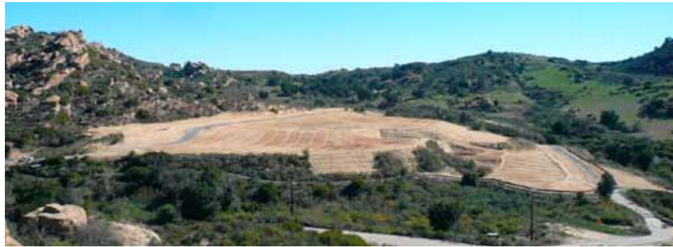
After. Components Test Lab III after demolition and hydroseeding
