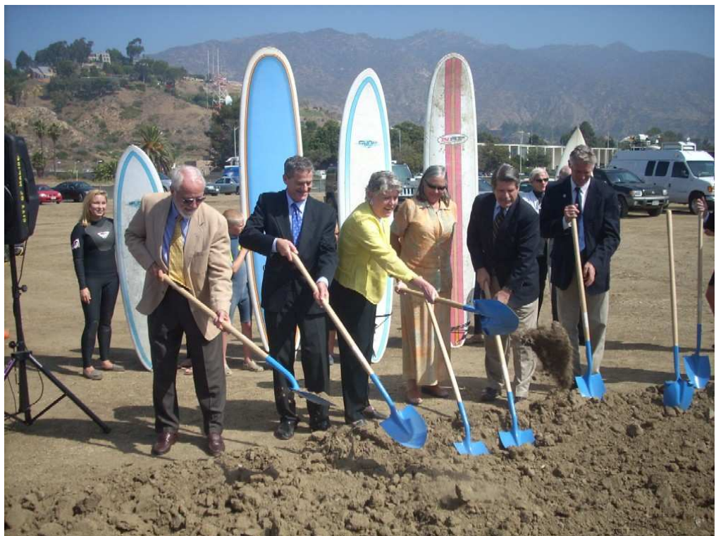
September 21, 2009 – Groundbreaking for Malibu’s Legacy Park. It will provide stormwater control, and include a public park and wetland restoration habitat.
