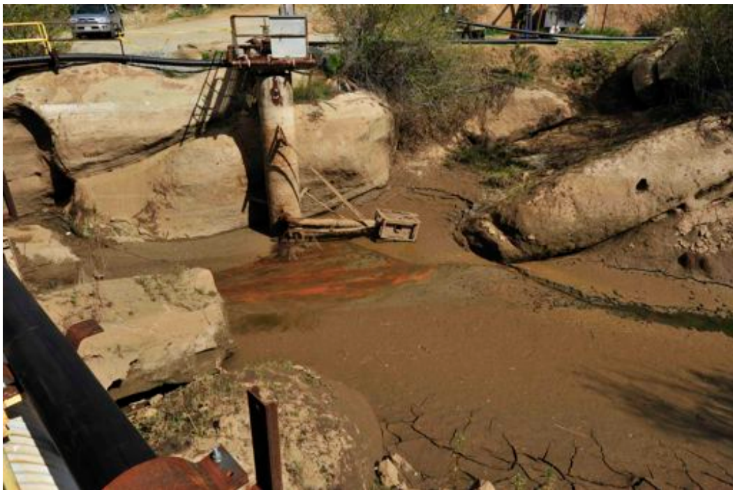
The pipes at this overlook were leaking and appeared to be the source of the discolored water below. These pipes are used to move water to AND from the pond, connecting the R2, Silvernale and other ponds with a system that move water both to and from these ponds.
