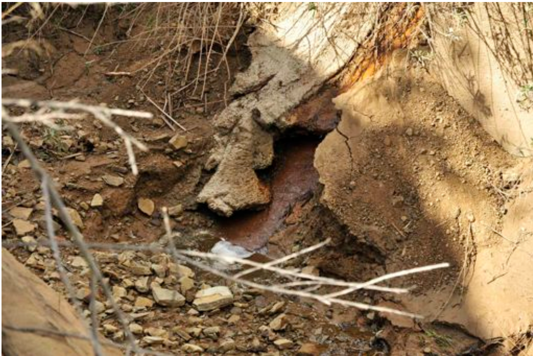
Foam observed at a second influent flow leading from what is believed to be the upper pond.
