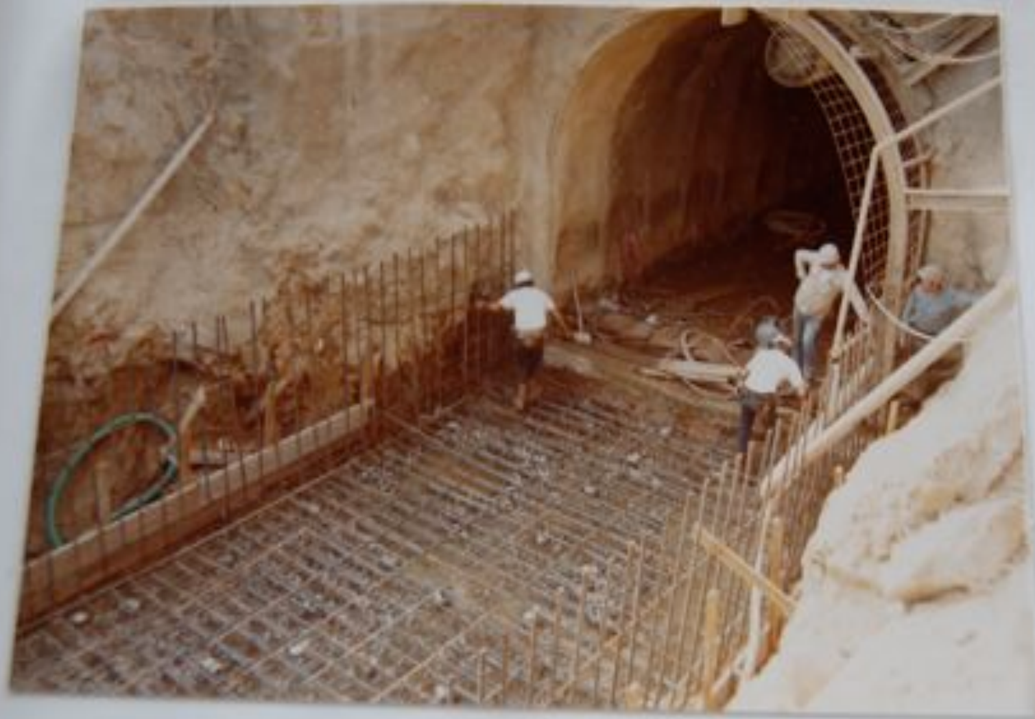
February 18, 1972 - Placing reinforcing steel for invert of open channel at the south tunnel portal. Steel set is at Station 10+03.
