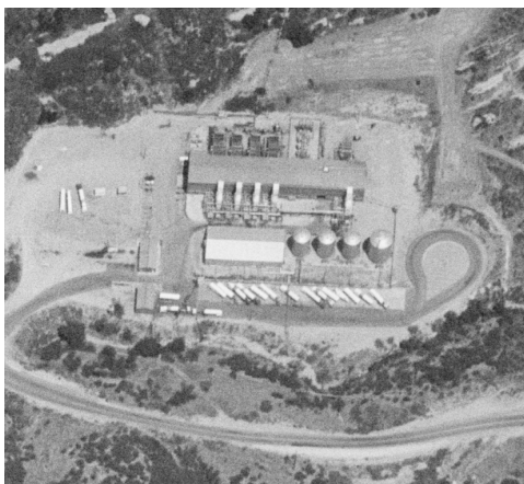
Former Liquid Oxygen (LOX) Plant
