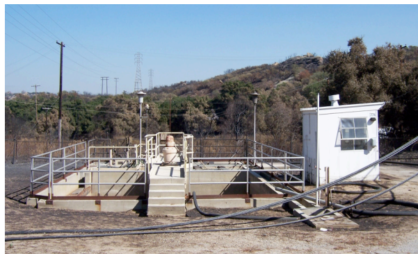
Sewage Treatment Plant
