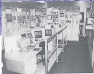
Small Components Test Loop (SCTL)
