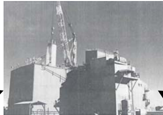
Component Handling and Cleaning Facility (CHCF)
