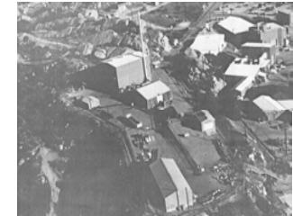
Radioactive Material Disposal Facility (RMDF)
